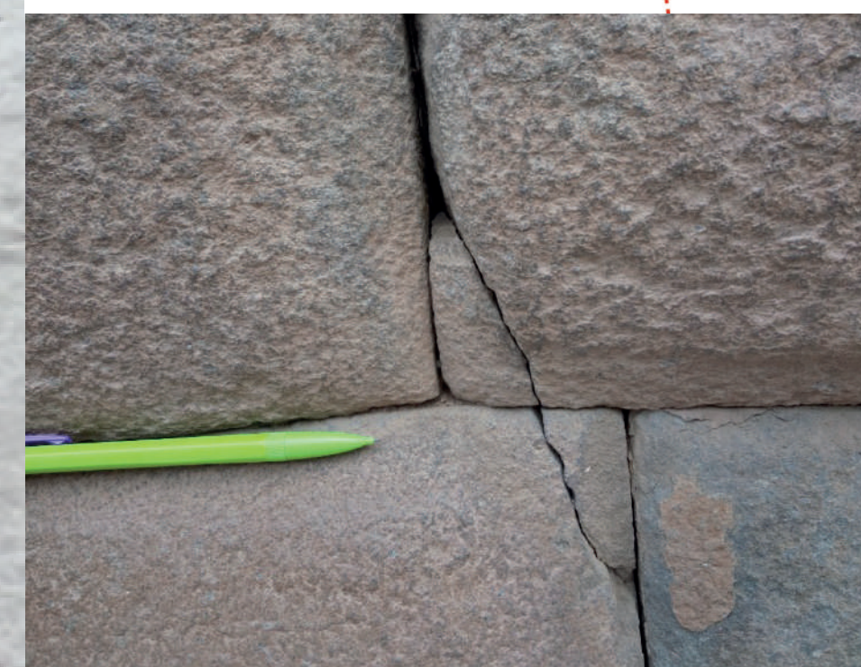
Fig.III Diagram of one of the most common type of EAE: the Dipping Broken Corner (DBC) with an illustrative example.
