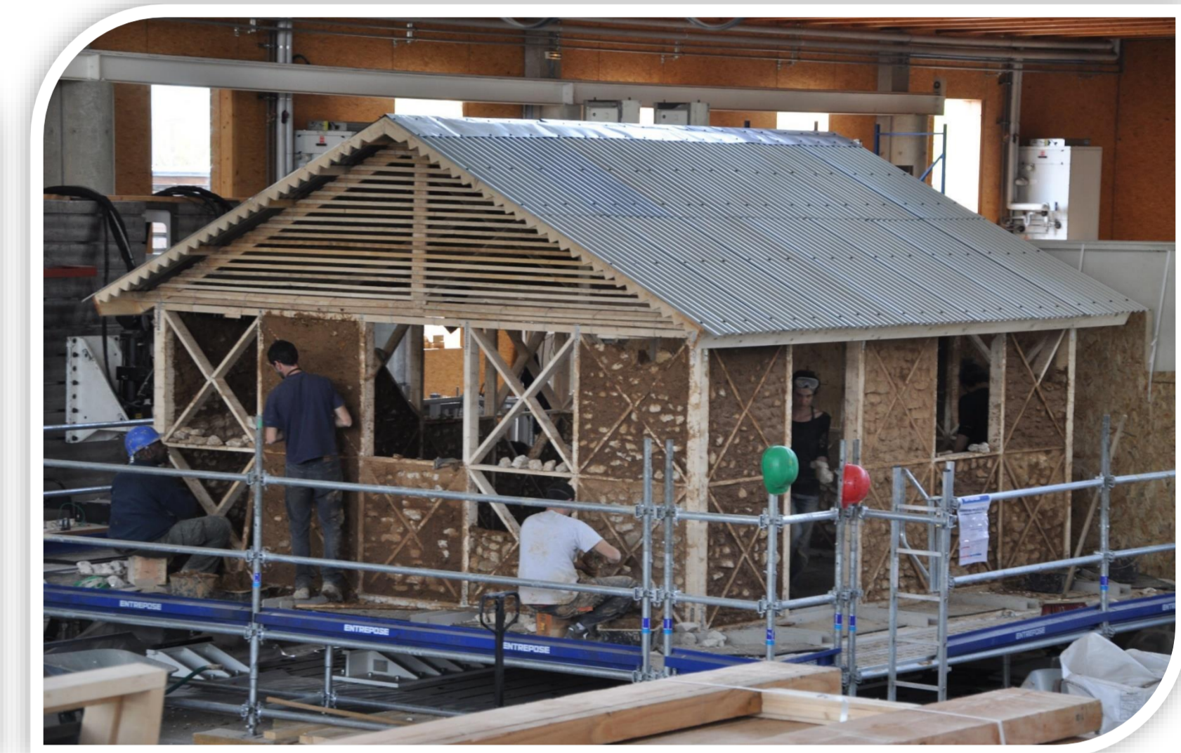
Fig.2 First prototype construction on shaking table in the ReparH project framework
