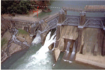
Shih-Kang Dam, Chi-Chi earthquake, 1999, Taiwan [Faccioli, 2008]
