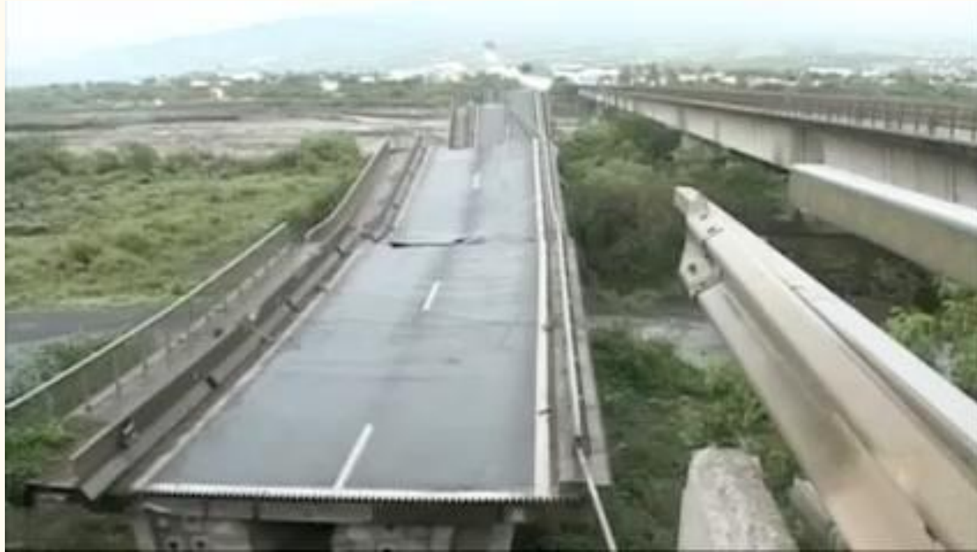
Collapse of one of the two RN1 bridges over the Saint-Etienne river during cyclone Gamède on Reunion Island, February 25, 2007.
