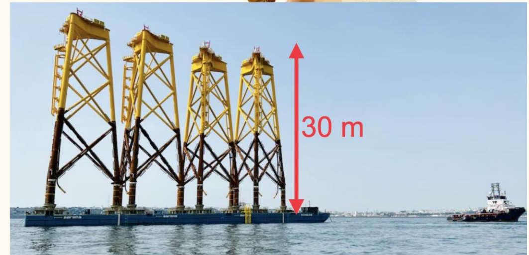
Arrival of the first four jackets for the future Saint Brieuc wind farm in the port of Brest
