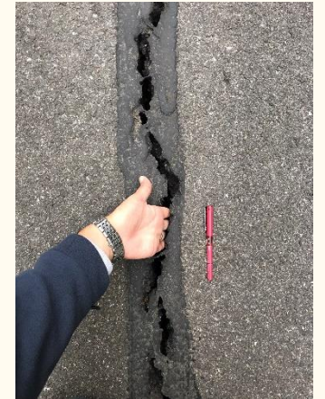
Desiccation waves during a drought episode at ground level under roadsides
