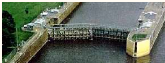
Lock gates (USACE, 2002)
