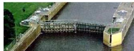
Lock gate (USACE, 2002)
